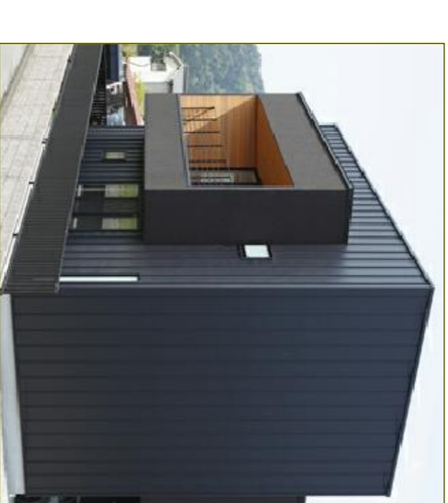
Reference Material - Zinc interlocking seamless cladding in two colours from manufactures palette as agreed with Planning
