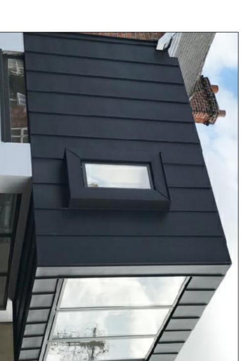
Reference Material - Zinc interlocking seamless cladding in two colours from manufactures palette as agreed with Planning
