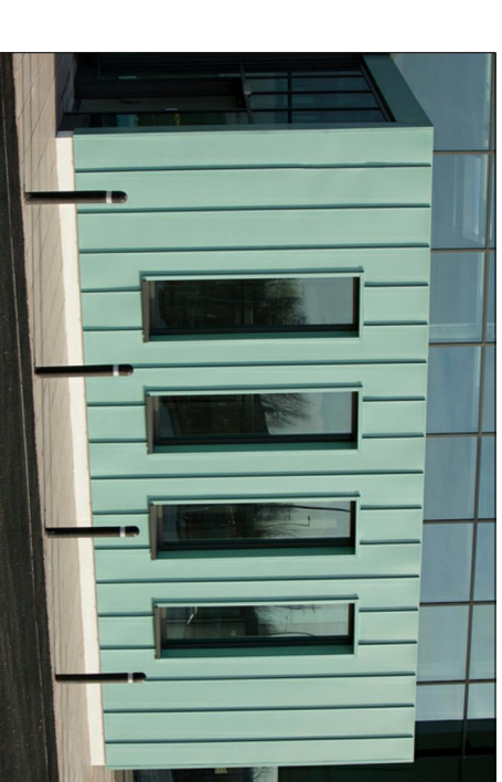
Reference Material - Zinc interlocking plank facade. Finish and colour as agreed with Planning at detail design stage.
